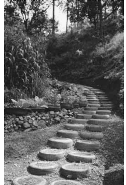
As part of their reconstruction efforts in the aftermath of Hurricane Mitch, the Honduran community of LaGranja Loma Linda used anti-erosion techniques to build this foot path.
